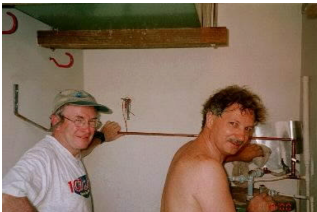
Jim, KP2L and W0CG working on plumbing.
