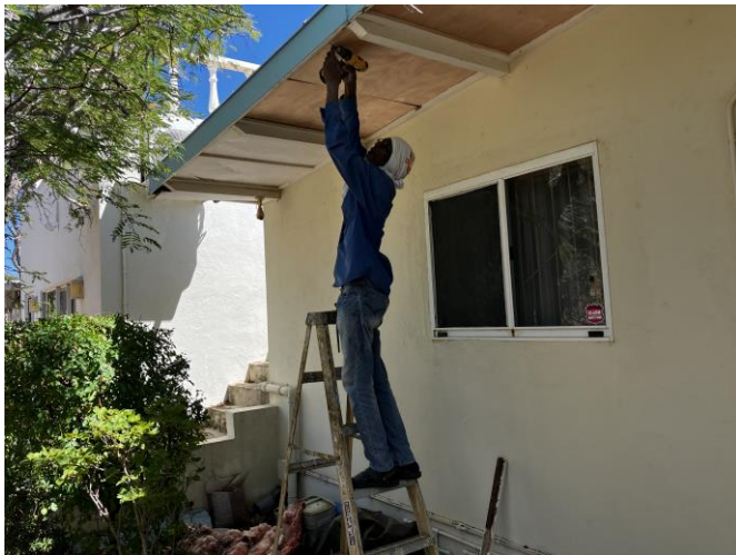
Ribert replacing soffit panels, 23 March 2026
