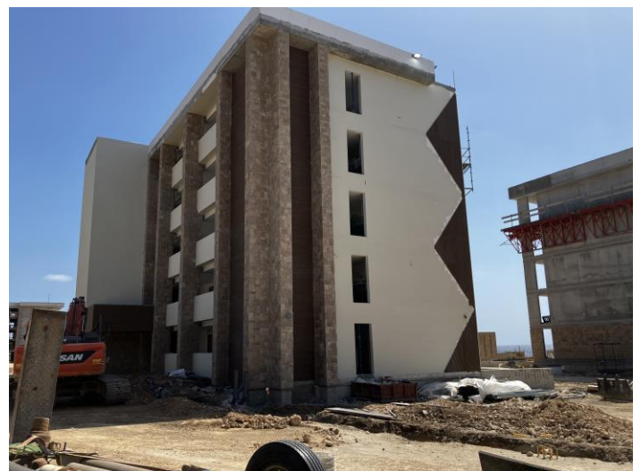
One of the six residence buildings taking shape, March 1, 2026.
