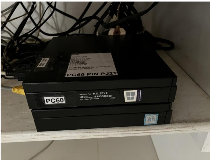
Windows 11 on top, 10 below; typical installation, this is at Station 3.
