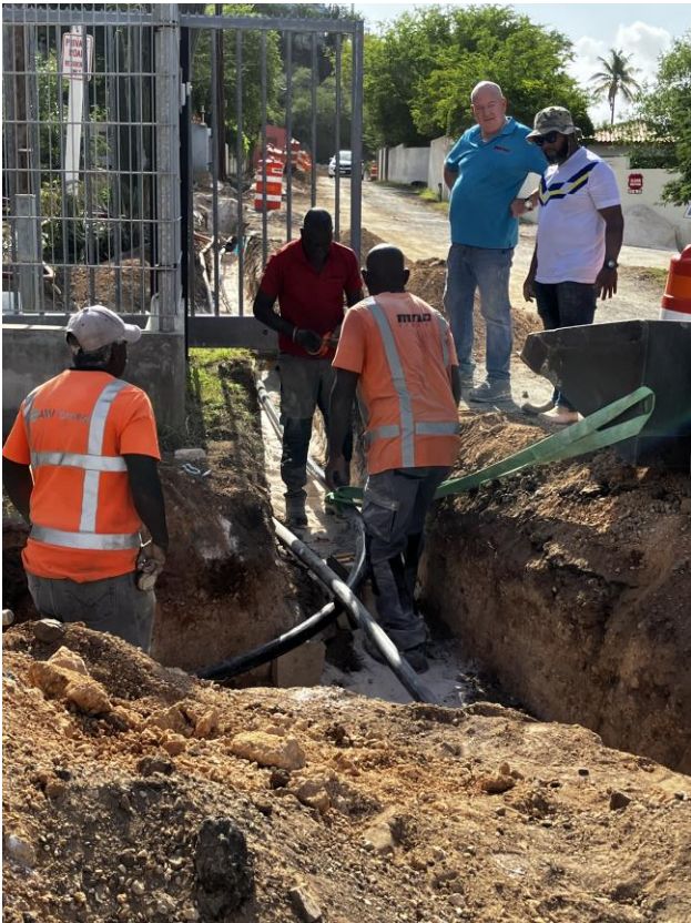
Legacy cables that have fed the neighborhood for 53 years, carefully unearthed.
