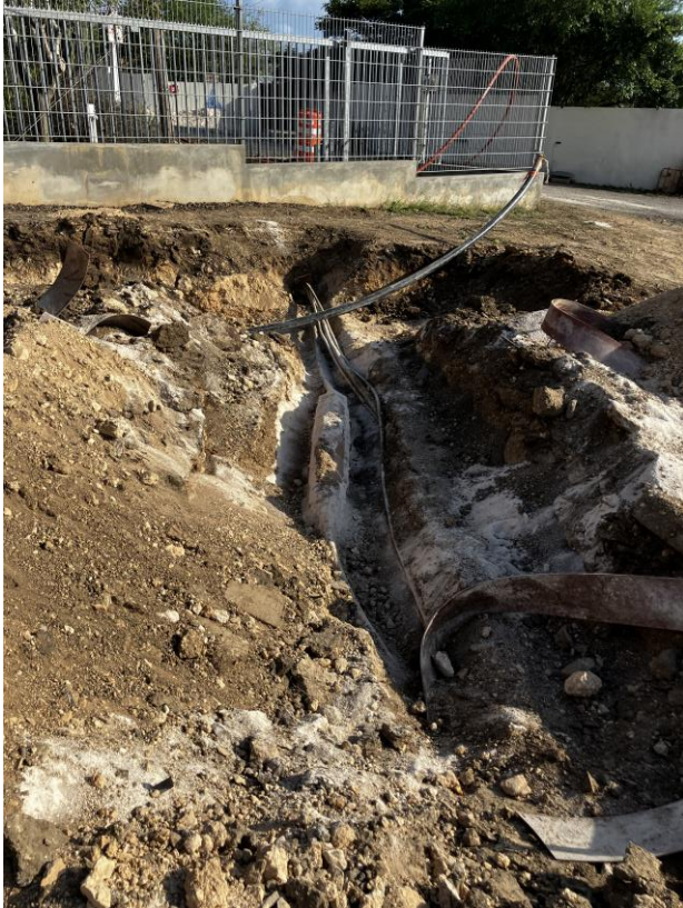
Legacy cables that have fed the neighborhood for 53 years, carefully unearthed.
