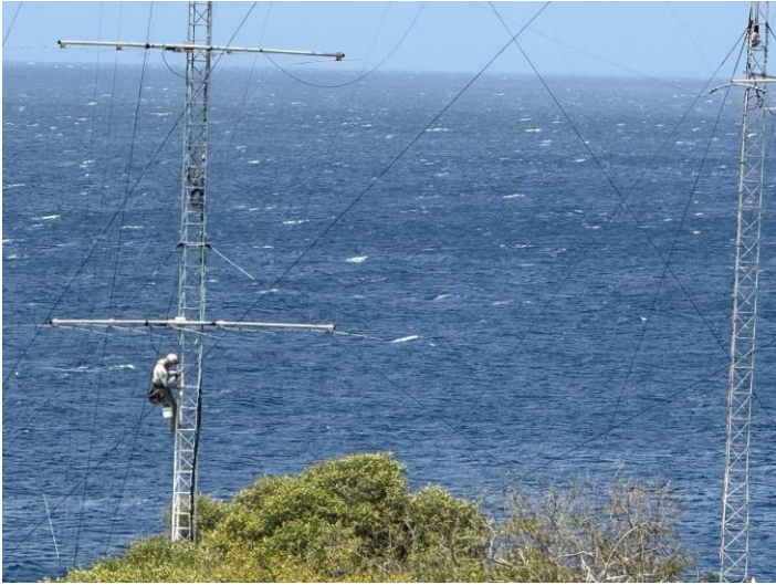
March 25, Geoff painting below the 10 stack (Photo W2APF)
