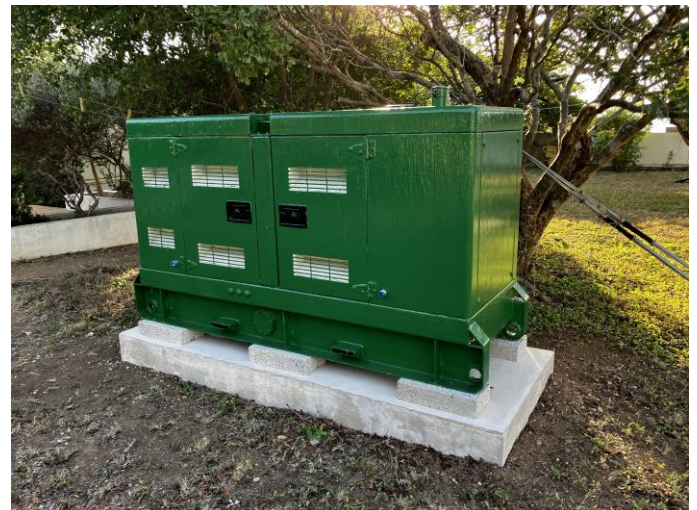
Signal Point powerplant in its final location, March 10.
