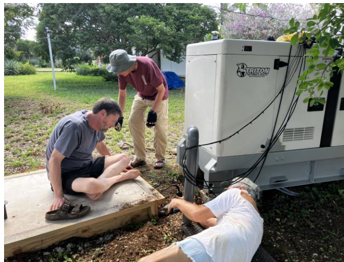
N7WA, K7TQ, and W0CG removing forms, February 17, 2025.
