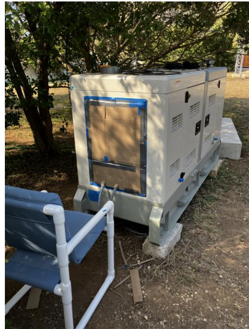
Generator masked off and ready for paint, March 4.
