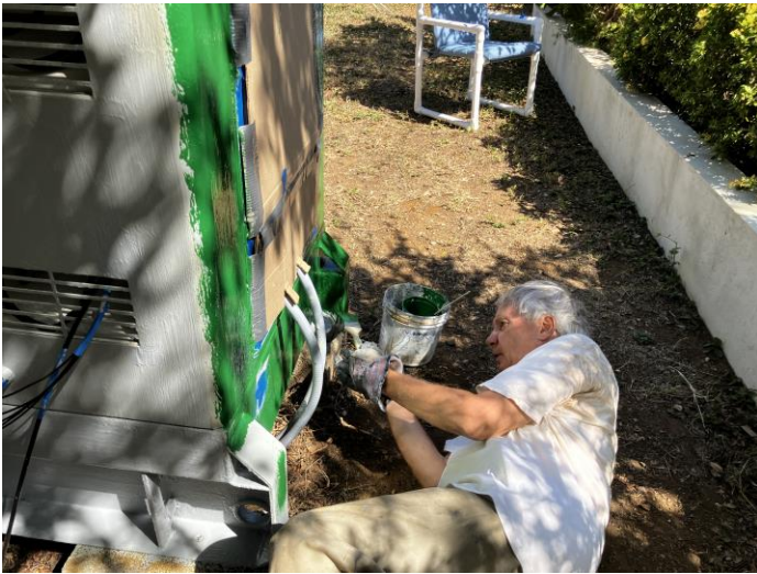
Working on the finish coat, March 6.
