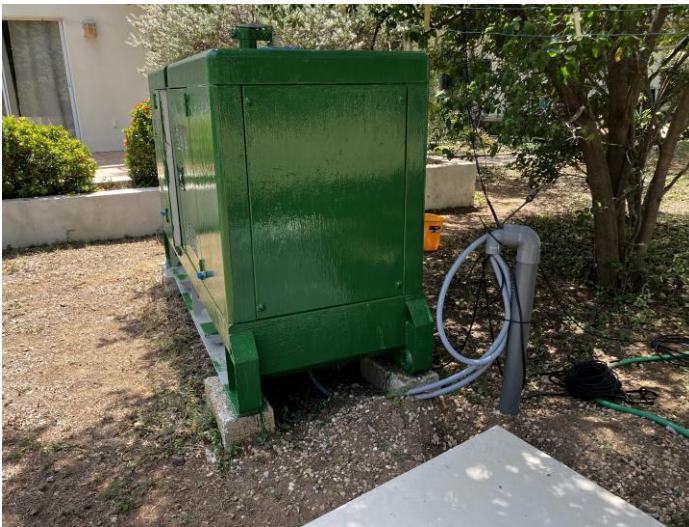
The completed paint job, March 6, 2025.
