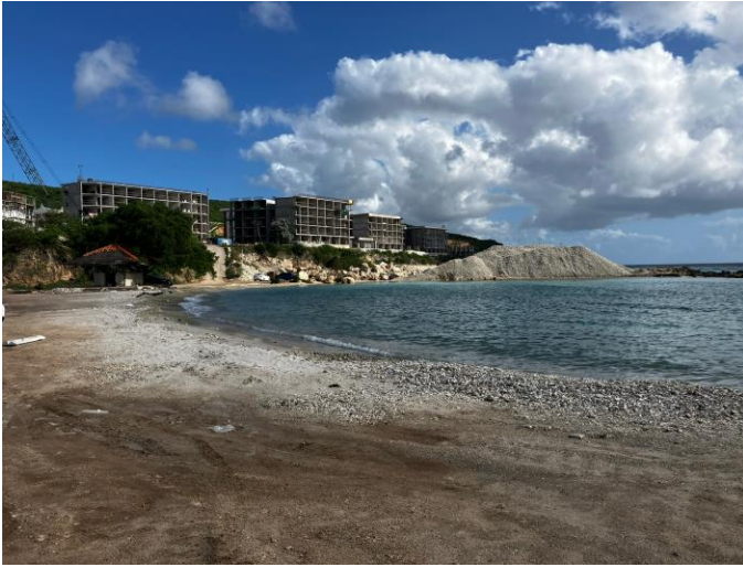
Progress on the Tui Blue hotel is very rapid now.
