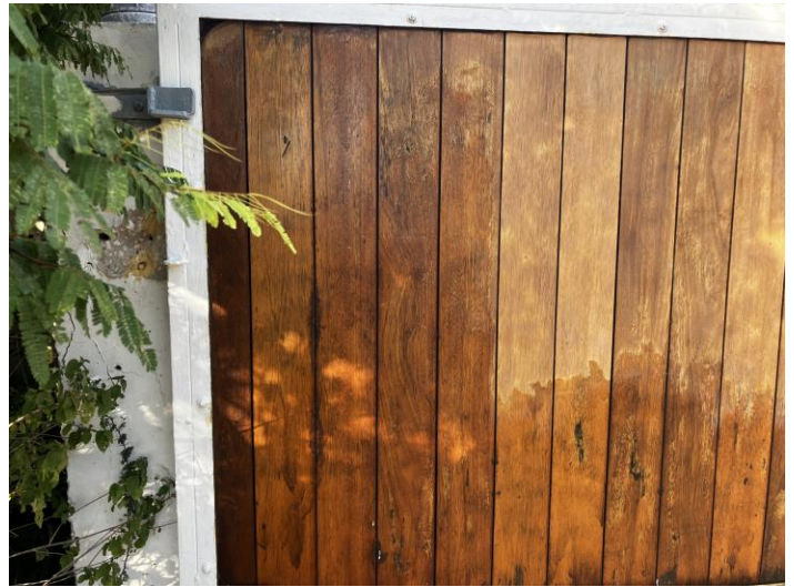
November 13: The part remaining to be sanded shows clearly here. Note the black stains in places. This maintenance will clear those up completely. Finishing this last part of sanding will take about five hours, believe it or not.
