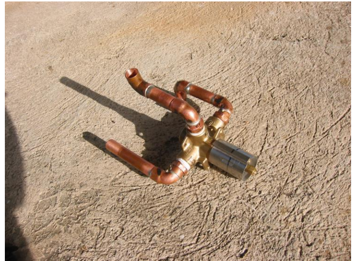
W0CG-fabricated shower control kludge ready to be installed
