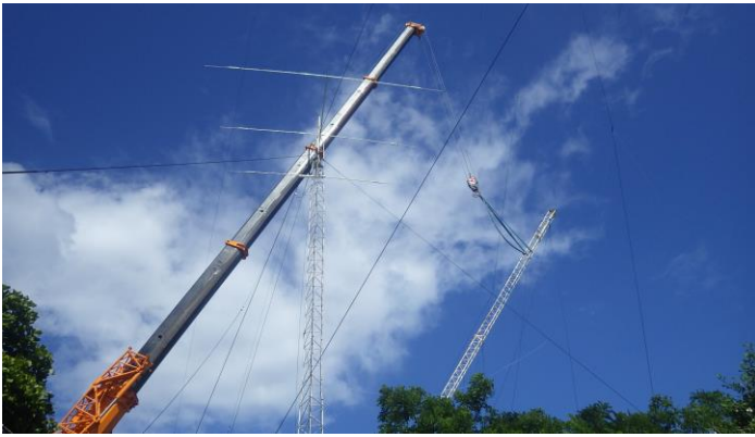
Easing the old tower to the ground.
