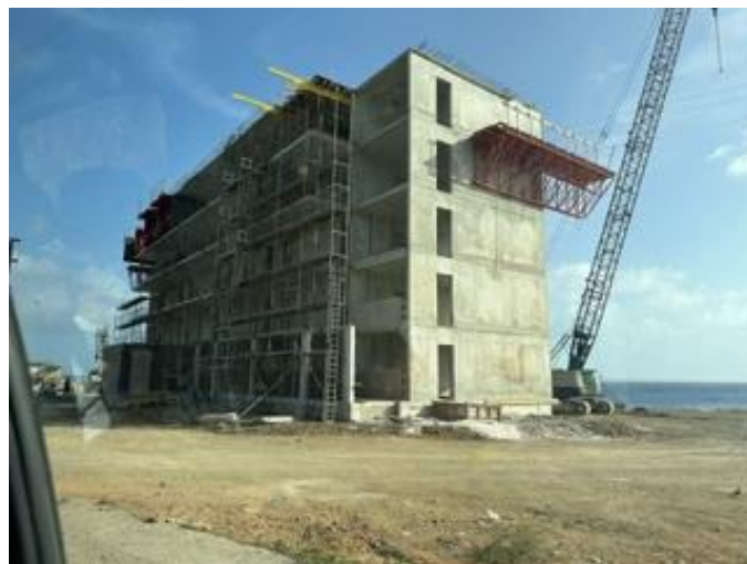
Building 1 at the new hotel (Photo PJ2BR)
