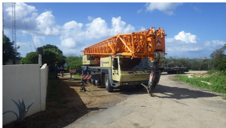
Setting up the crane outside Signal Point's west wall, December 4, 2018.
