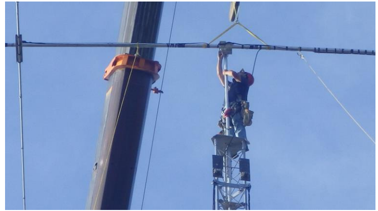
Very brave and capable, W3YQ maneuvering the new 40 meter yagi onto the new tower and mast. Tim donated all of his time as well as his travel costs!
