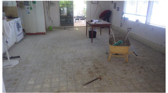
October 6 after we removed the old tile floor.
