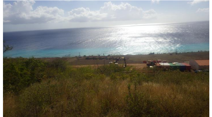
Foundation footer forms in place below
