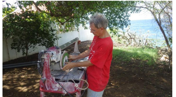
Geoff setting up the tile saw prior to cutting pieces.
