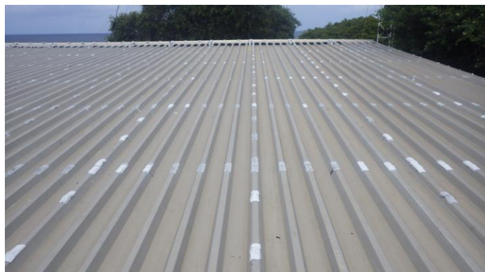
The bright white tapes are the new ones. Thus far I've installed about 200 feet of tape.
