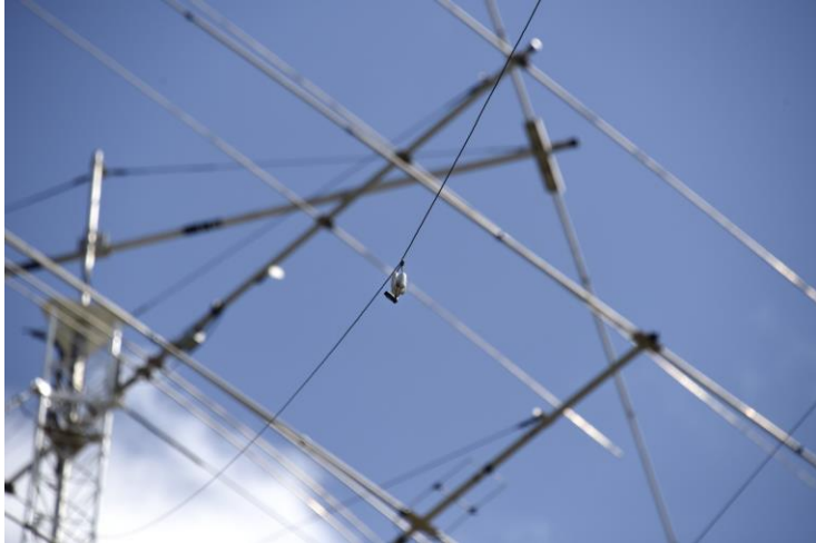
Broken insulator rope (center, in focus) (Photo K8ND)
