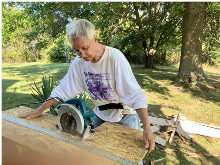
W0CG cutting patch pieces for the chimney
