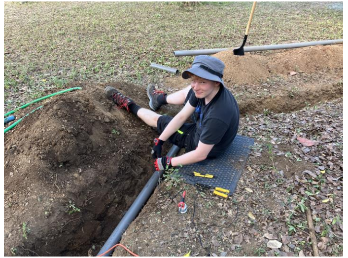
DL3ON patching and soldering broken radials
