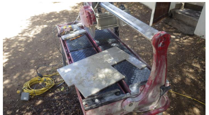
One of ~350 custom cut tiles, March 1, 2015
