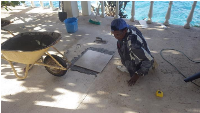
Ribert sets the first of 657 tiles, February 28, 2015
