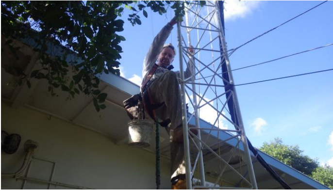
W0CG in the tower painting gear
