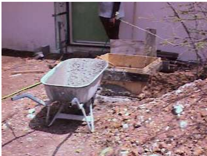
Pouring the base for the US/JA tower, June, 2001
