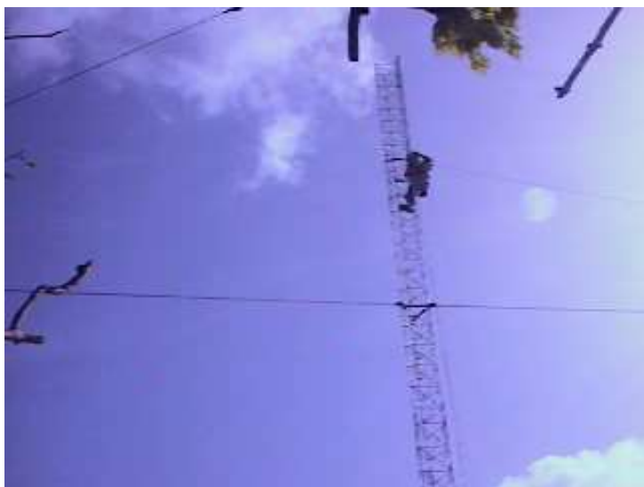
W0CG building the Europe tower, July, 2001
