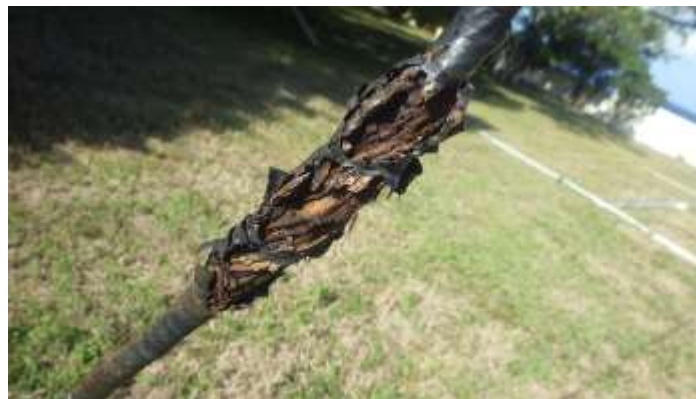
This severely damaged Philly big grip completely crumbled apart in my hand.
