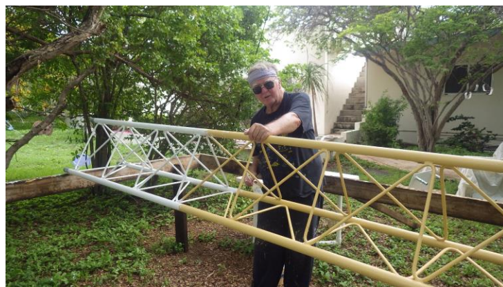
Mid-October, WI9WI putting finish epoxy on one of the new sections.
