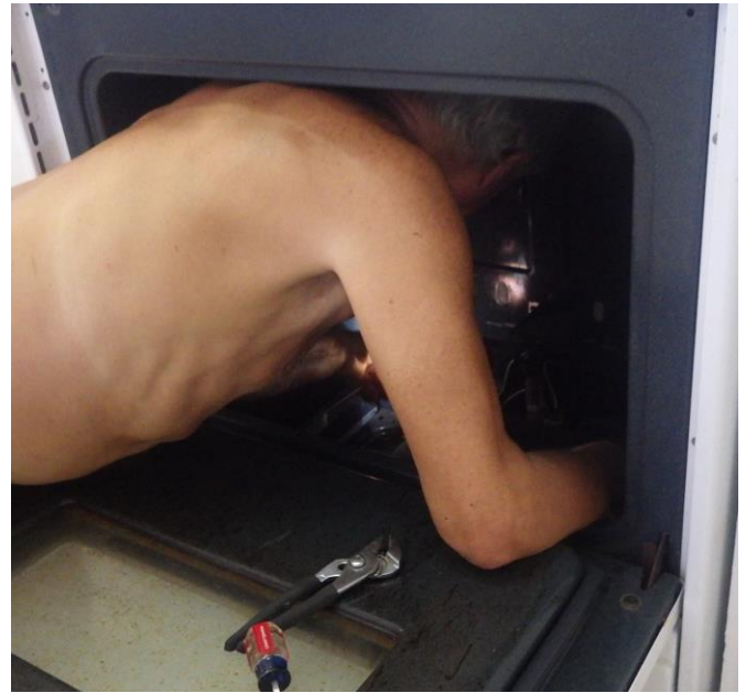
Fixing the oven igniter, icky and dark and awkward
