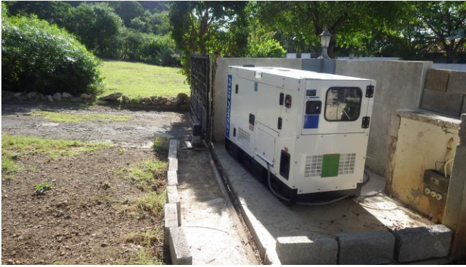
Dirk van Daam's generator: a 25 KW diesel
