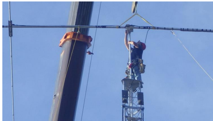
W3YQ atop the new tower fitting the new 40 yagi to the mast
