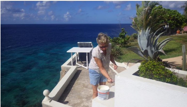
Freshening up the top coat of paint
