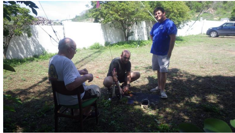
Rich (W3ACO) directing, Levi (KG5XR), and Connor (W4IPC) as we assembled the antenna permanently without the transformer.
