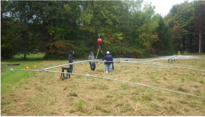
Prepping the lift of a giant four element 40 yagi to go to the top.
