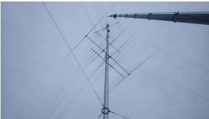
The top of four tribanders being positioned at almost 180 feet. If you've never climbed, you can't imagine how frightening this appears to the climber.
