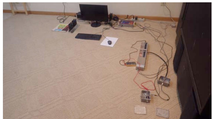
PJ2T remote station in mock-up in Ohio
