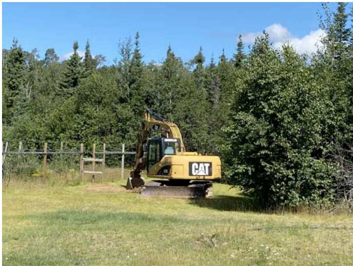
At the new VE3CX QTH: Tower Construction
