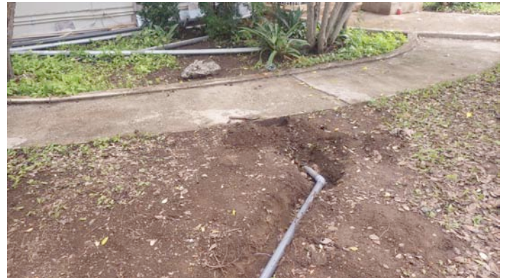
Fiber conduit under the back sidewalk (March 2022)
