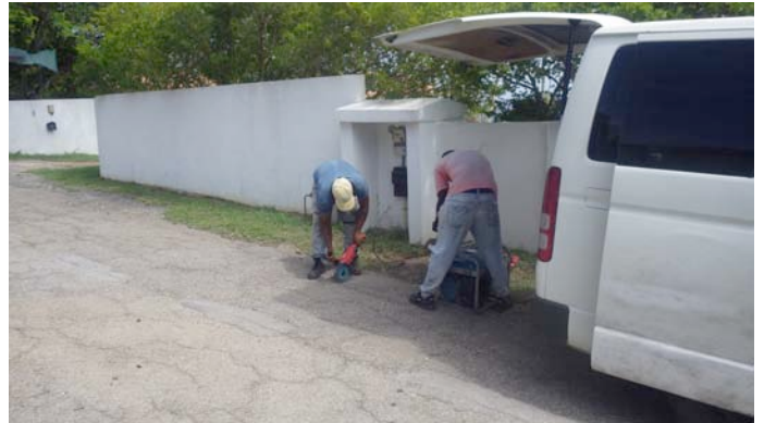
Beginning the cut through the pavement
