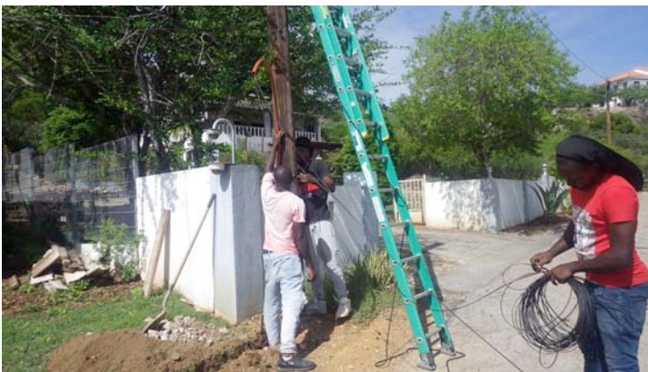
Routing the orange conduit containing two fibers up the utility pole.
