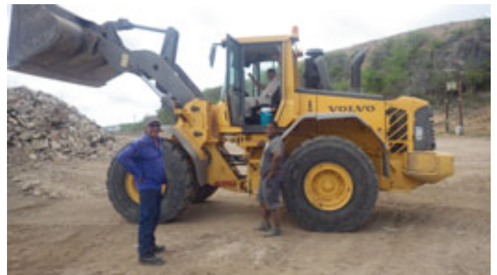
Celebrating the last pile of dirt removed
