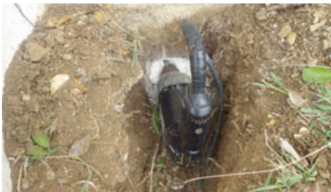
Hole through wall from street to backyard for fiber
