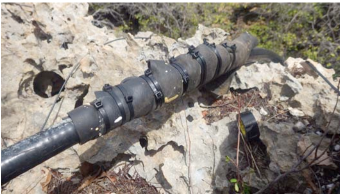
The relocated Ridge feedline, protected from abrasions at the cliff edge
