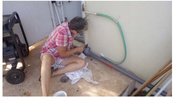
Dorothy starting the exterior priming of the new plumbing.
