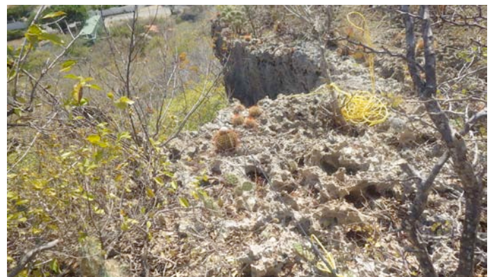
The new RG-6 feedline (center of photo) from the feedpoint and down over the cliff, with Signal Point's front wall visible far below.
