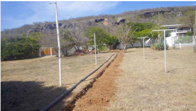
Just prior to burying the 75 mm conduit.
