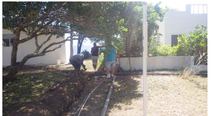
Above, trimming up the dig at the conduit split point.
