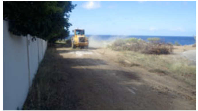
Pre-clearing land for construction, February 9, 2022
