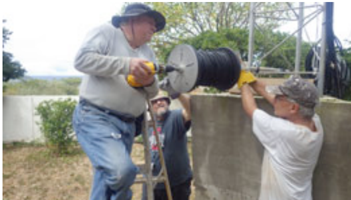
W8WTS winding, W0CG serving as a shaft collar, and K8ND as traveling capstan as the cable winds in rapidly.
