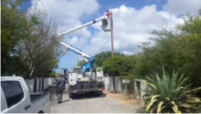
Contractors installing fibre optics lines in our Coral Cliff neighborhood, February 10, 2022.
