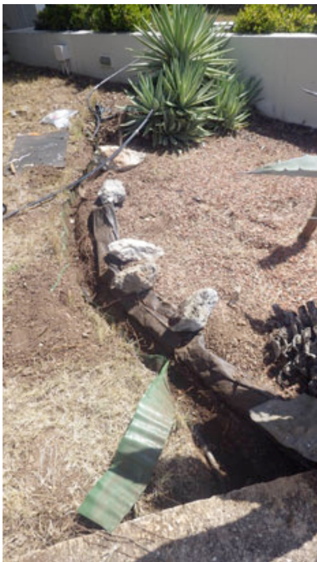
The blocked line was somewhere along this 25 foot hand-dug ditch.
