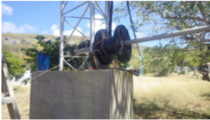
Spooling out 1000 feet of cable to the 4 square
