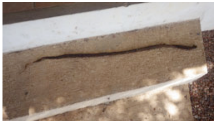
The two foot long root bundle that I pulled out of a 3/4 inch plugged irrigation line.
