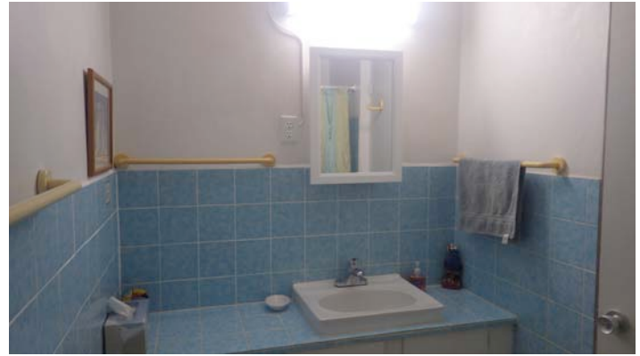
New cabinet, light, and outlet in West Bathroom
