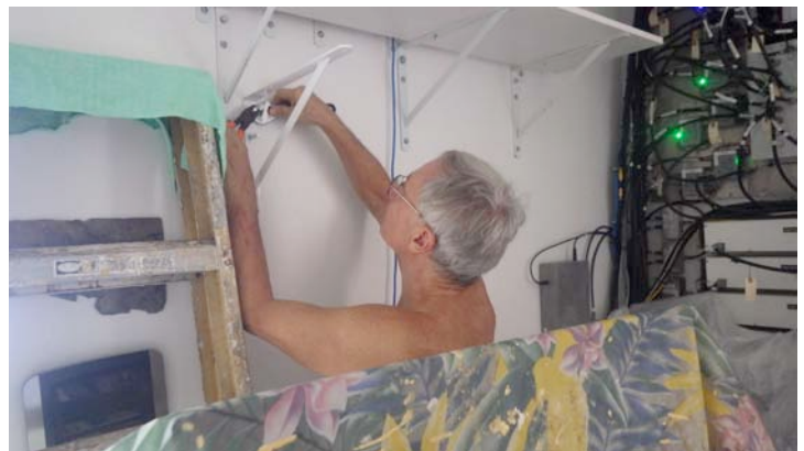
Installing masonry anchors for the KPA-1500 power supply shelf
