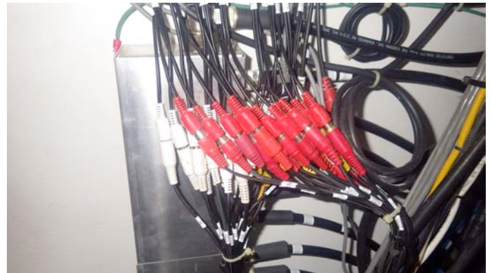
DC antenna selection lines to select from...
