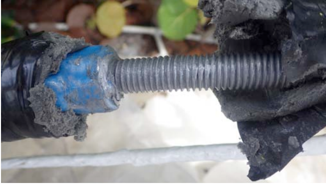
Threads on turnbuckle in perfect condition underneath our putty/tape weather seal.
