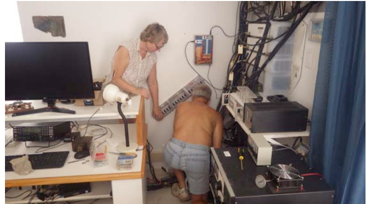
Drilling mounting holes in the concrete for the 1 x 18 box
