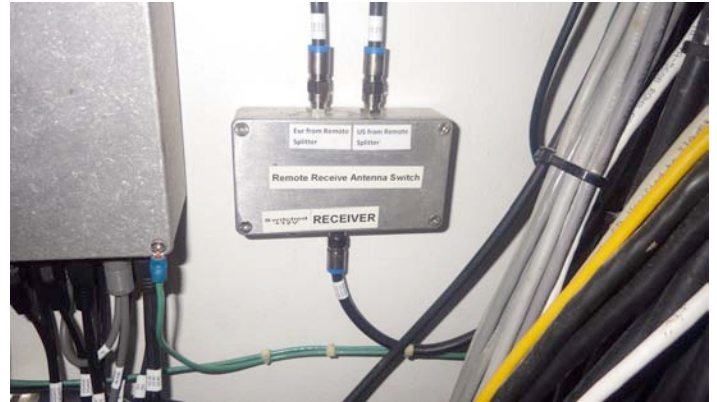
N7IR remotely-controlled RX antenna selection box
