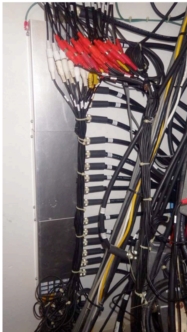
1x18 homebrew remote station coax switch
