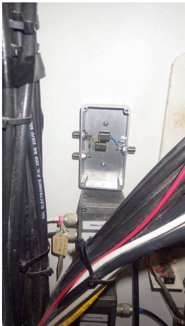
An N7IR RX splitter with its hood up
