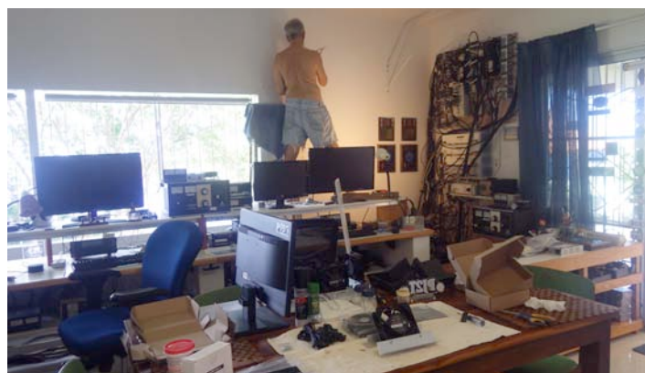
October 14, Geoff installing the top shelf for the enhanced remote
