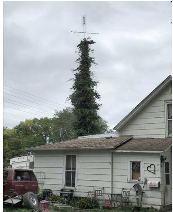
Reinforced tower in Redwood Falls, MN
