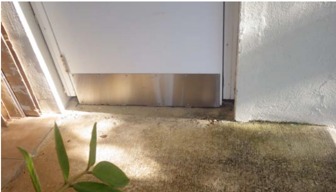
New stainless steel kickplate on Step Closet.
