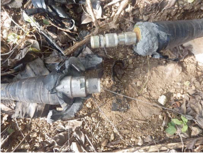
Ridge hardline opened across the road
