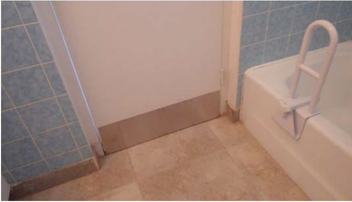
The safety bar donated by KB7Q in the West Bathroom
