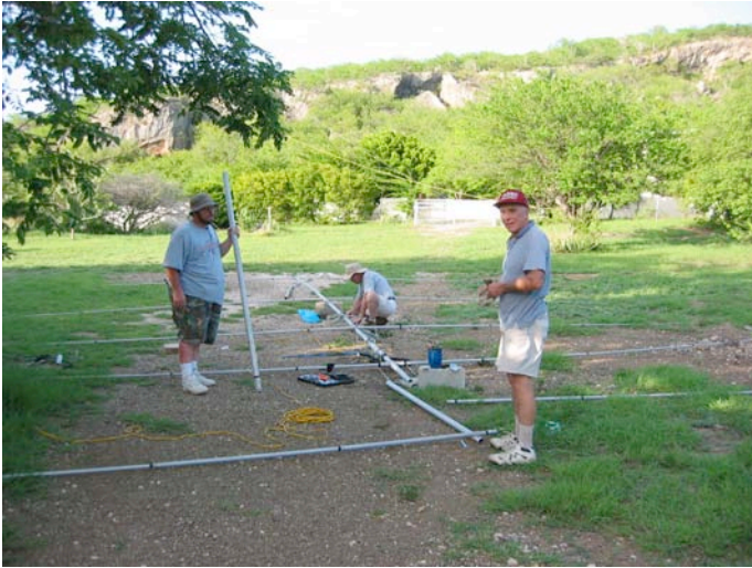
Here's my view from the tower just prior to hauling the 20 meter beam up the tram rope and reinstalling it, totally renewed and salt-proofed.
