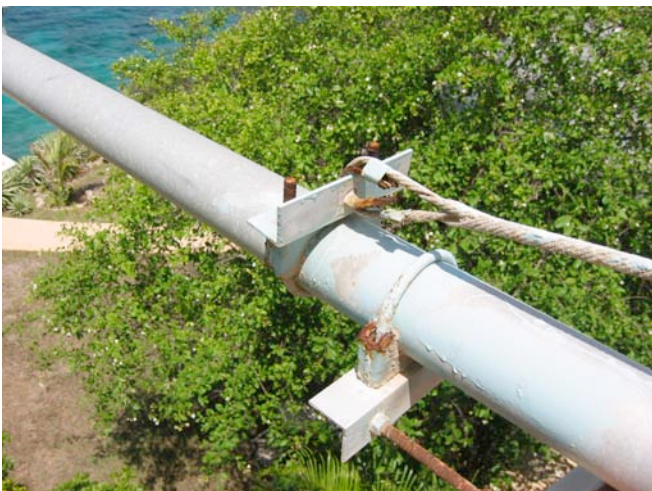
The antenna rebuild project continued into 2007. We took down all the yagis from the US/JA tower, resting them on the railings of the roof terrace. Here are some corroded parts on the boom of the 15 yagi prior to replacement, July 11, 2007.
