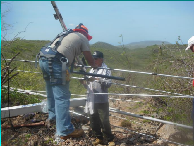
NR0X and W0CG installing elements.
