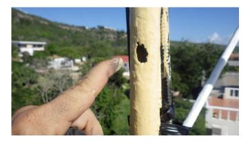
This was underneath a wrap of tape that was holding up feedlines. We have now learned not to use tape on tower legs, and it has nearly all been removed. This hole is not as heinous as it looks, because tubing is still very strong with this small proportion of its circumference lost. As you see, this hole has a coat of epoxy primer. The next day I coated it with epoxy paint and the day following installed a leg splint. There is no need for concern, as this will hold up for many years.
