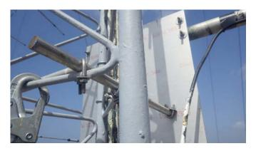
One of the most unique aspects of the new tower is the stainless steel thrust bearings that were obtained by N0YY. Two of these have served well on the US tower for four years, and two more are now installed on the Europe tower. Also pictured (right) are the stainless hardware on one of the guy brackets and the stainless cable thimble (painted grey).
