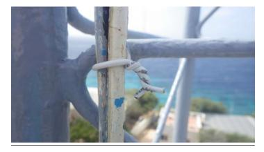
Instead of taping to the legs, all feedlines are fastened to the bracing pieces – not the legs -- with a wrap of insulated #12 solid copper wire. This will never corrode, and it minimizes contact with the tower.
