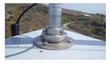
As you see, the bearing and the very thick-wall aluminum mast at the top of the 100 footer are in excellent condition at nine weeks. I'll update you on other design features of the new tower in future issues. We can be very proud of the design, engineering, and construction of this great new PJ2T asset.
