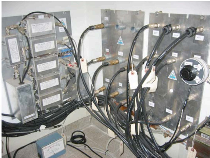
The coax entry bulkhead and filters when everything was shiny new, September, 2002.
