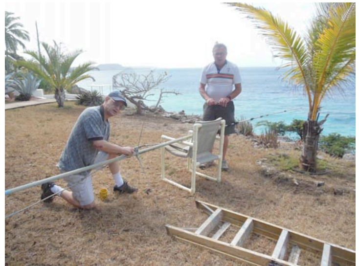
VE7AM and N0KE working on the Ringo Ranger, March 27, 2013.
