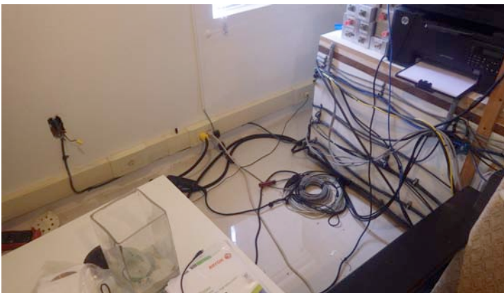
Installing permanent power to the ASUS router.
